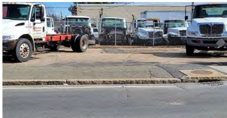
Is this a sidewalk or a parking lot? This creates an unsafe condition for both pedestrians and drivers.
